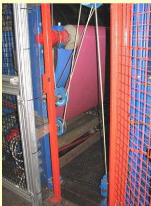
General view of the area with the access gate open
